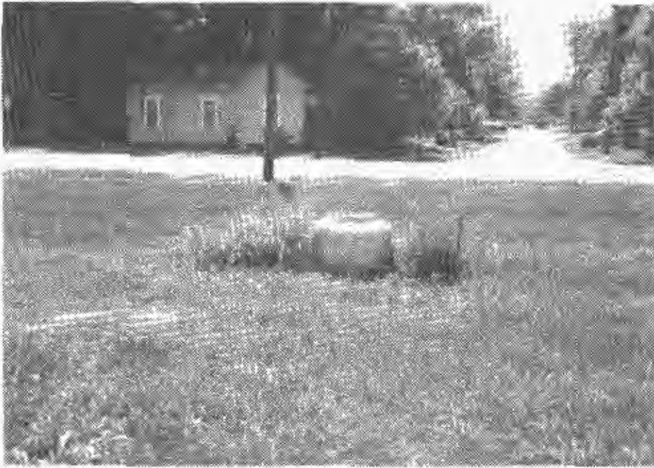
LIVE OAK - DRAINAGE WELL NO. 3
