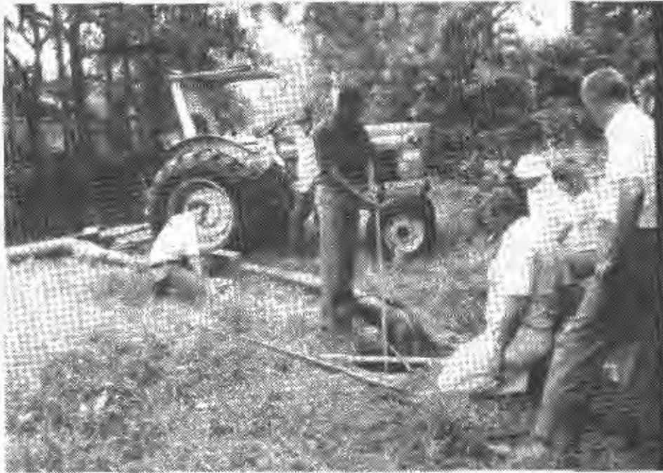
LIVE OAK, FLORIDA PUMP TEST ON DRAINAGE WELL NO. 33
